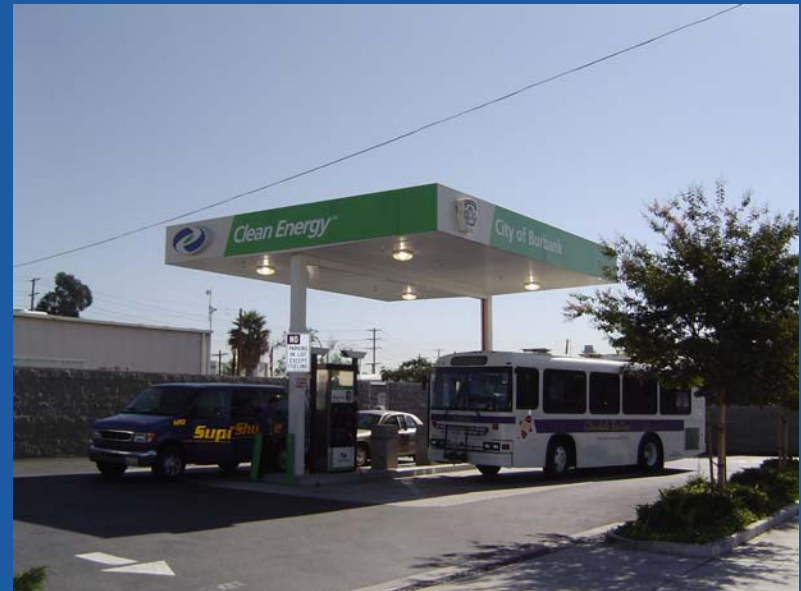
City of Burbank CNG Station
